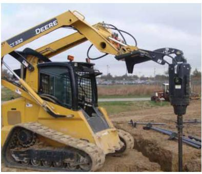
Long reach skid mount used to install helical anchors.
